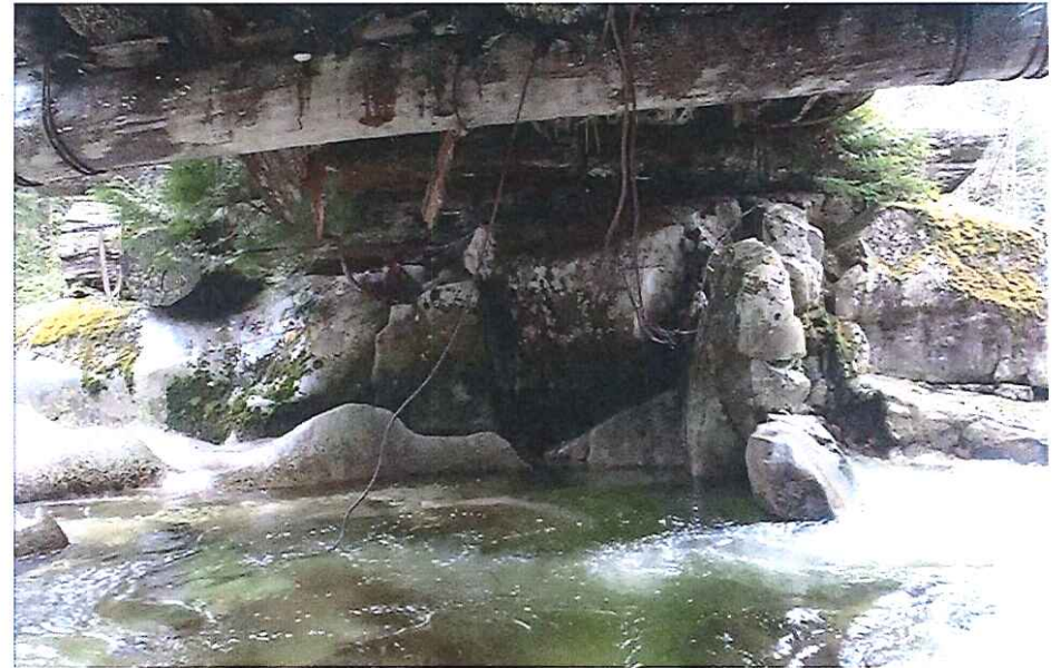
CK2394 Right Abutment
